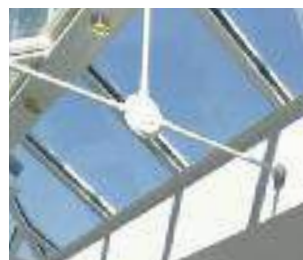
Tie bars - create the classic Orangery roof space with ornate, non-structural tie bars.
